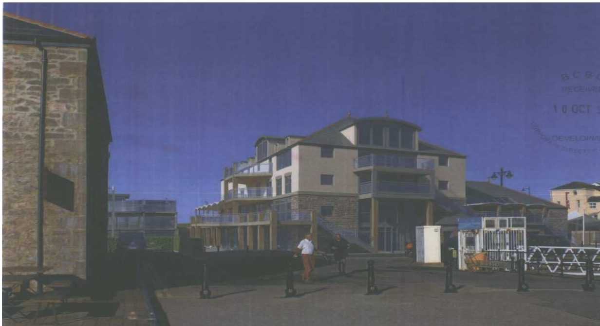
Figure 6: View of the building from the northern corner of the Jennings Buildings
